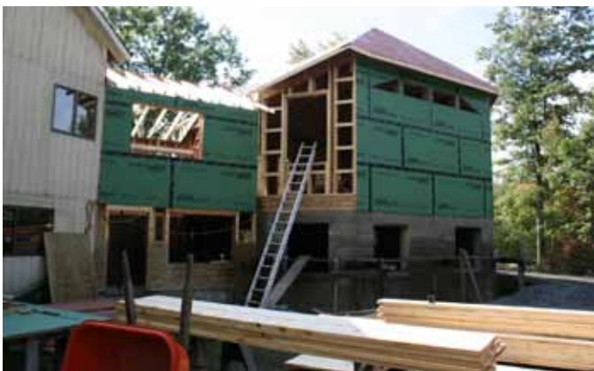
The walls for the upper story go up. The walls are framed with a double row of 2x4 studs, so that they are 9 inches thick and form no thermal bridge. They will be insulated with cellulose.
