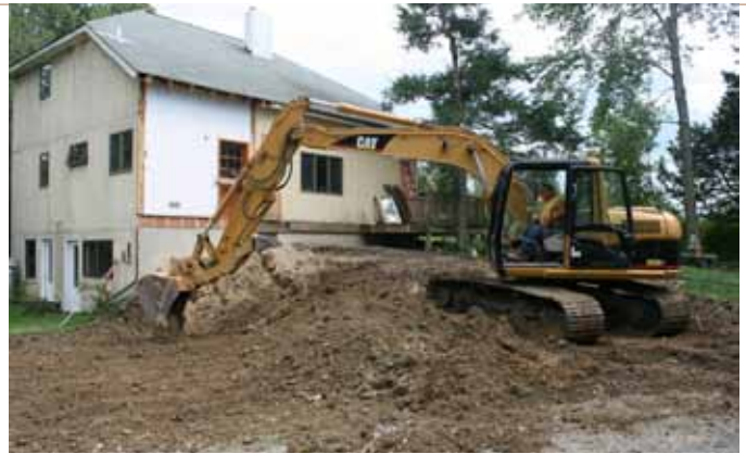
Excavation for the new wing
