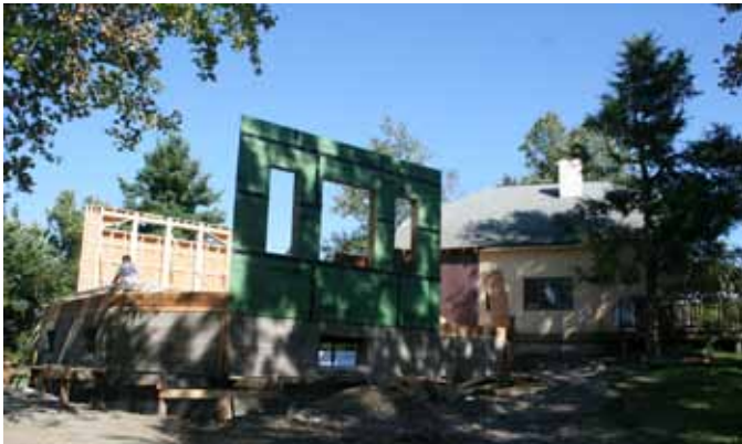
The walls for the upper story go up. The walls are framed with a double row of 2x4 studs, so that they are 9 inches thick and form no thermal bridge. They will be insulated with cellulose.
